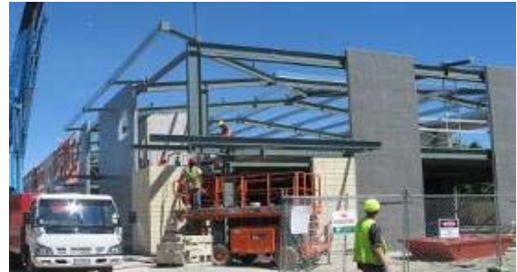
Construction of new TiDA facility
